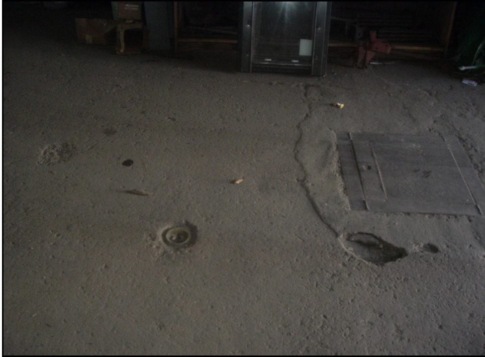
Photo 31: View of square access panel of possible UST/vault located at 1645 Warner Street.
