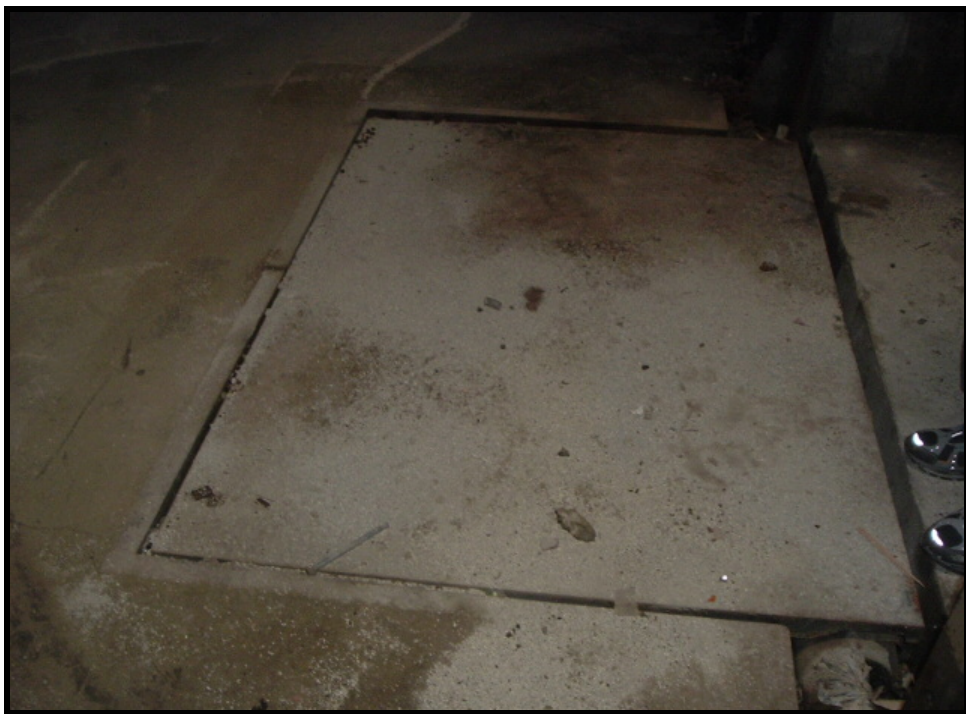
Photo 20: View of possible UST/vault metal plate cover at the 1601 Warner Street Warehouse.
