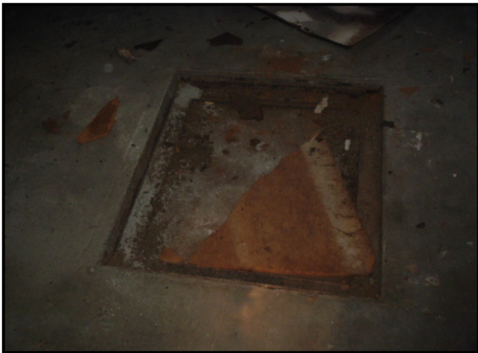
Photo 22: View of access panels of suspect UST/Vault at 1629 Warner Street Western Unit warehouse.
